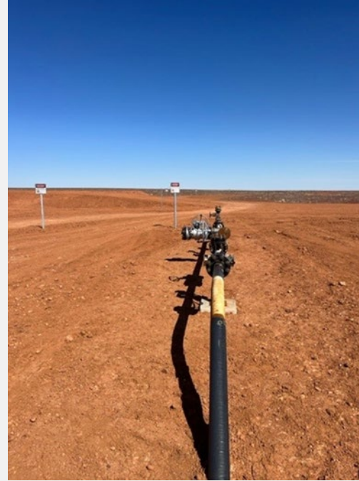
Figures 4 to 6: Yarrow Pipeline Completed. Pipeline predominantly laid underground with certain points above ground where necessary.
