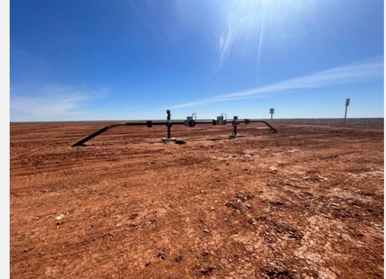
Figures 4 to 6: Yarrow Pipeline Completed. Pipeline predominantly laid underground with certain points above ground where necessary.
